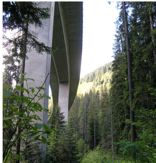
Fig. 23. Westbound I-90 viaduct crosses high above the Denny Creek Trail. This method of freeway construction, more common in the Alps, allows free movement of wildlife and greatly reduces the impact on the landscape, as well as reducing avalanche and rockfall risks to motorists.
