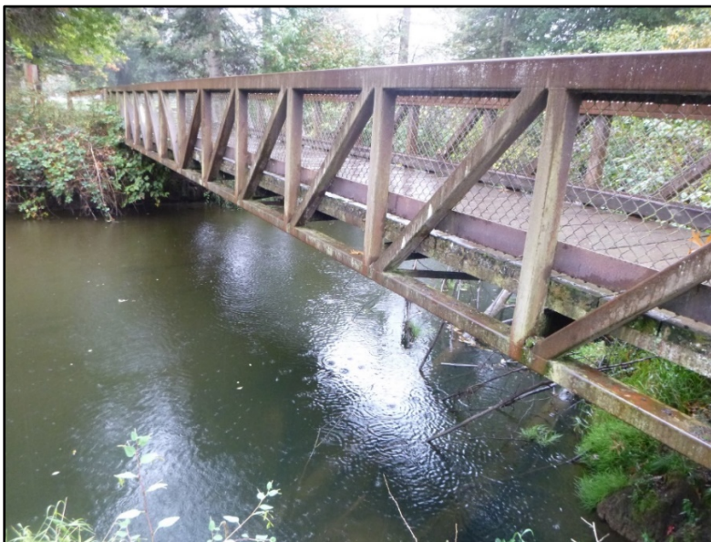
Photo 4. Pedestrian Trail Crossing Issaquah Creek in Reach 1
