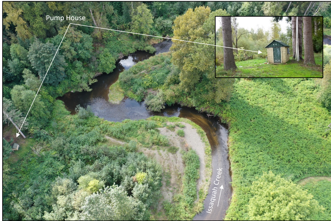
Photo 19. Existing Pump House in Reach 4
