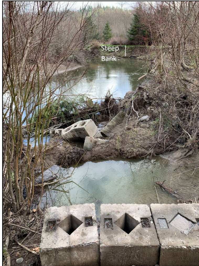
Photo 12. Pickering Ditch Failed Pedestrian Bridge (Photo Taken 2/26/2020)
