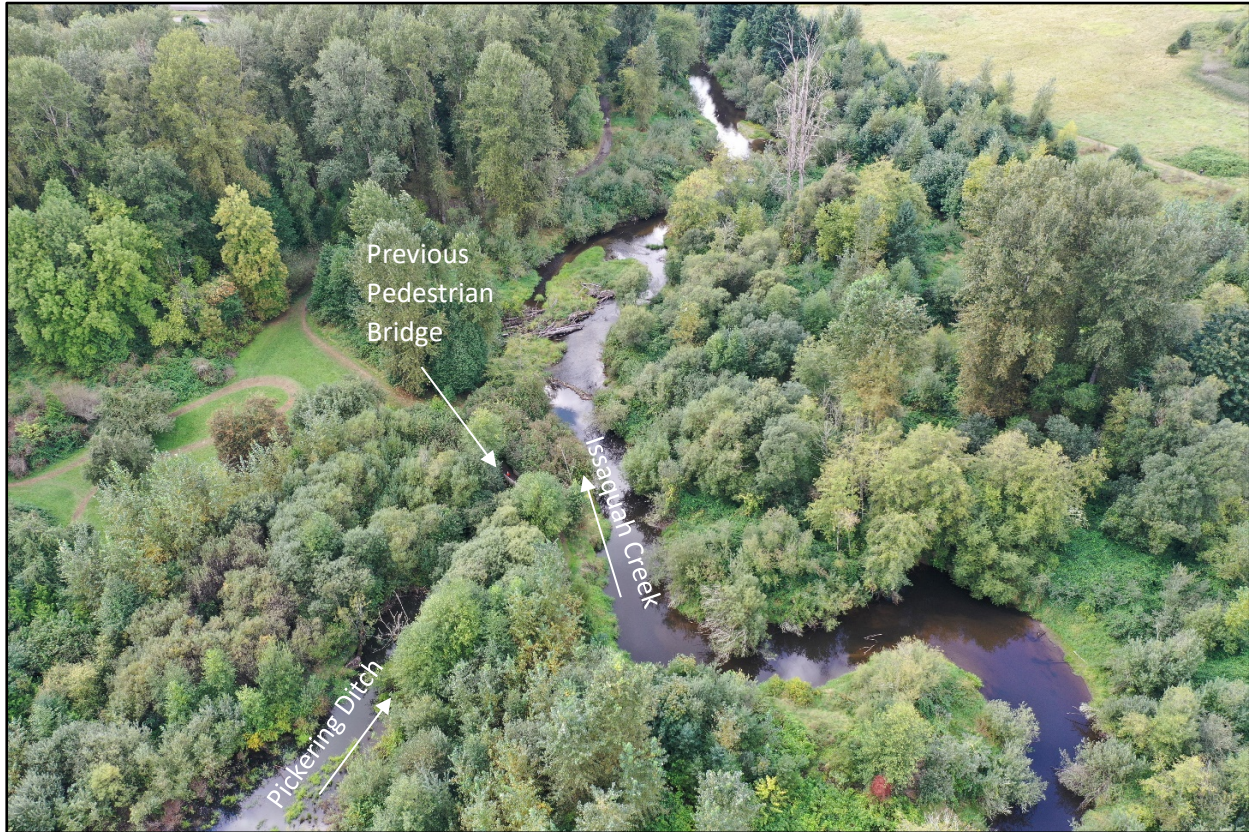
Photo 10. Reach 2 – Pickering Ditch
