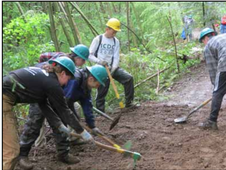
A new 5-mile trail on Mailbox Peak is under construction
