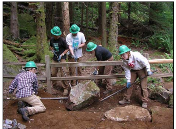
Mountains to Sound Greenway field crew members Michael Martinez, Martin Geier, Ryan McDonnell, Natalie Gough and Jackie Ford do some heavy lifting to build a rock turnpike on the Little Si Trail just outside North Bend. Greenway crews and volunteers completed a major renovation and improvement project at Little Si this year.
